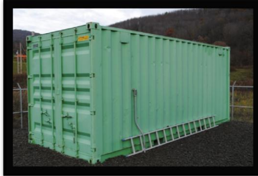
Shipping Container Metal Bldg
