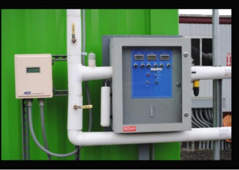
NOVA 41270QN4CW Oxygen and Methane Analyzer 8000
